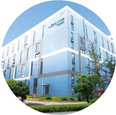
Jinan, China GMP Facility
