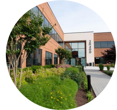
Maryland, USA, GMP Facility
